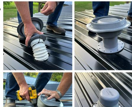
you cut the hole the size of the screw flange you can sit it down against the furring strips and attach with 4 or more screws. There are prepunched holes the whole way around the screw flange so you have a hole wherever you need it.
