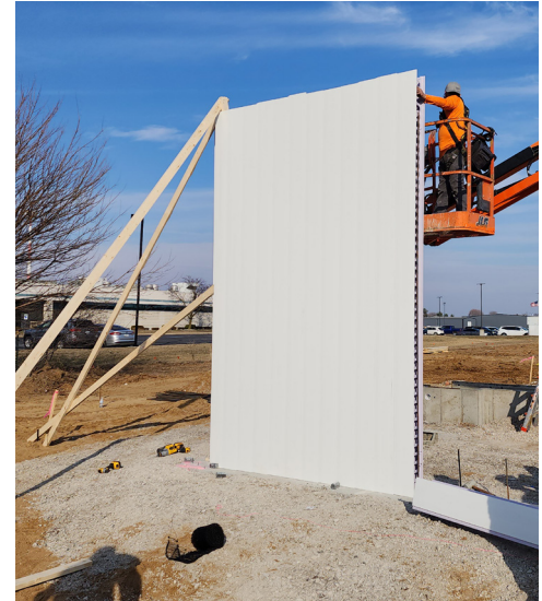
Ensuring Panel is Seated Properly
